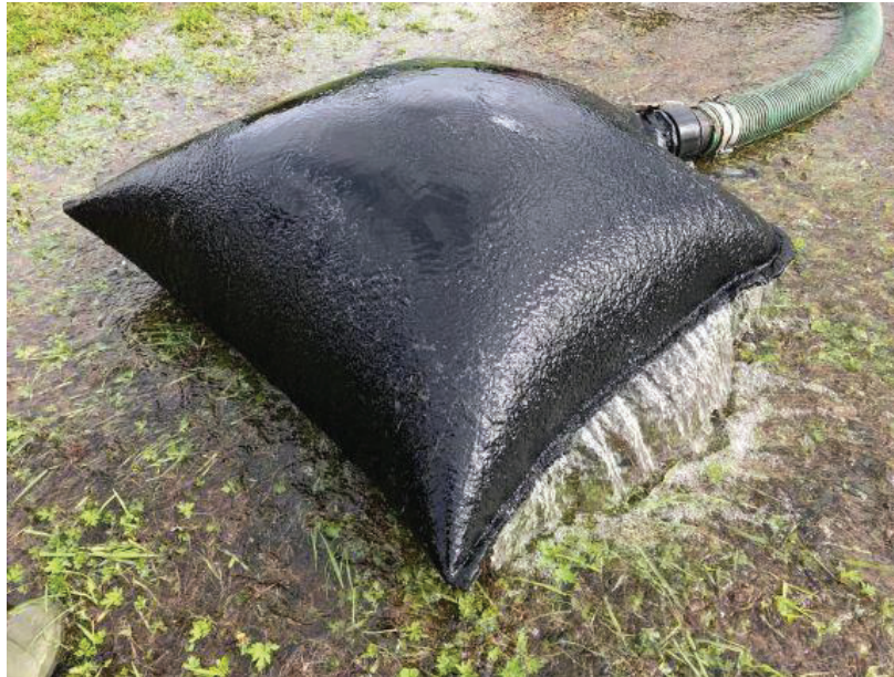
Figure 4.4: Dewatering bag ( https://www.murlaconline.co.uk )
