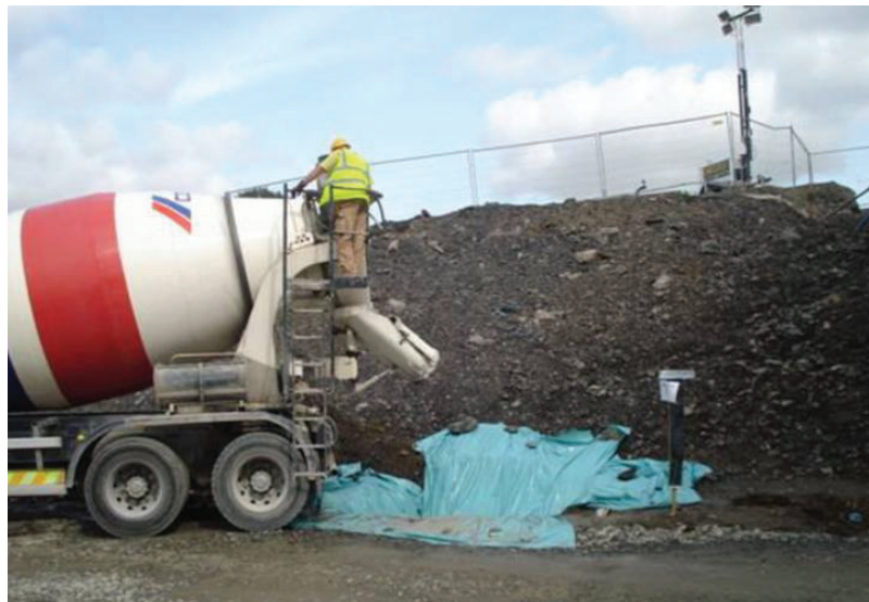
Figure 4.5: Concrete wash-out area with impermeable liner (TII)
